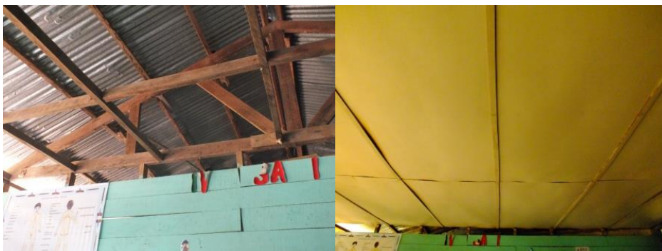
Photo N°3.- Before and after
