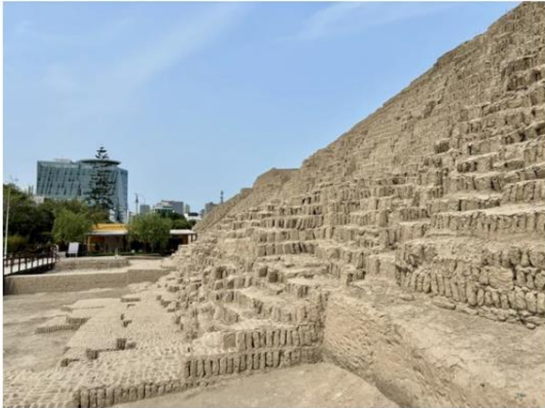
Huaca Pucllana adobe and clay pyramid built from seven staggered platforms sits in the Miraflores district of central Lima, Peru. CYNTHIA MCLEOD/TORONTO SUN torsun
